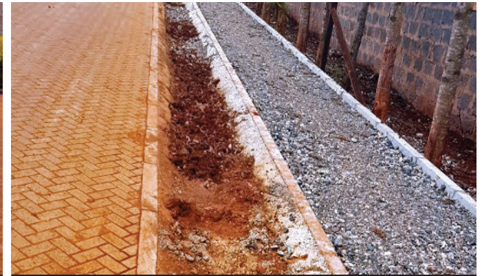
Pavement & Drainage Works
